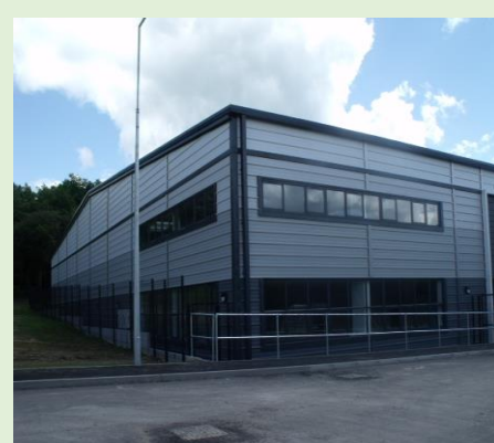
T54 – Plot 5c TWC starter unit – Operational
